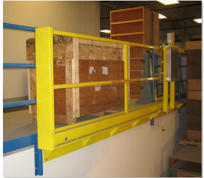
Automated Horizontal Sliding Mezzanine Pallet Gate
